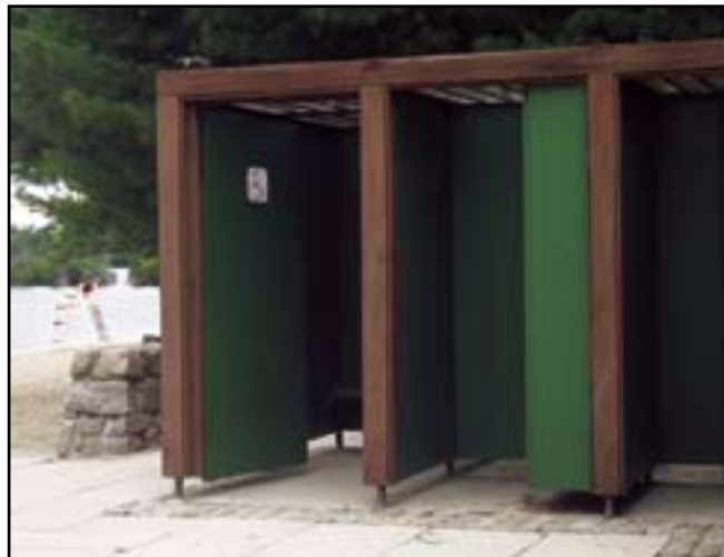
Accessible Change Rooms – Tour of Providence, Rhode Island / photo credit: Donna Rodman
