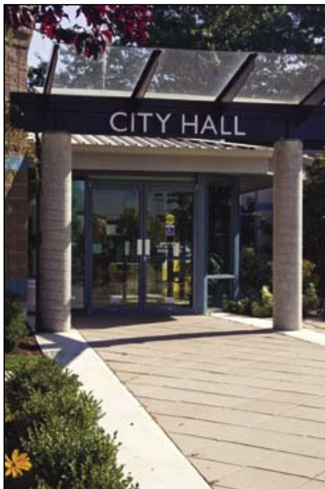
Accessible Building Entrance, Pitt Meadows City Hall, Pitt Meadows, B.C. / photo credit: Manfred Wuensche
